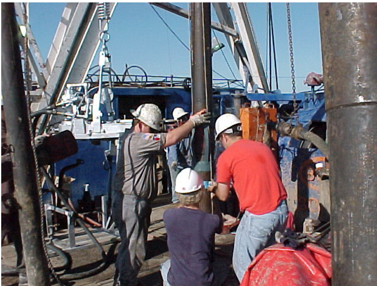
Figure 7.3 – Installing a Band Below a Centralizer
