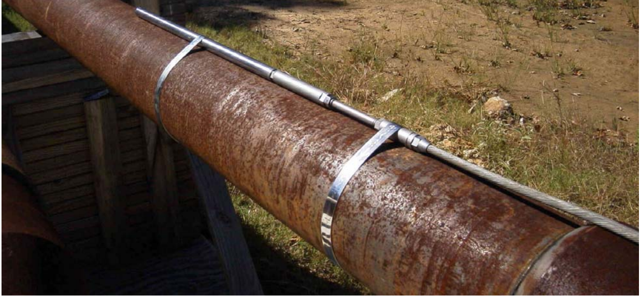
Figure 5.2 – First Strapping Method
