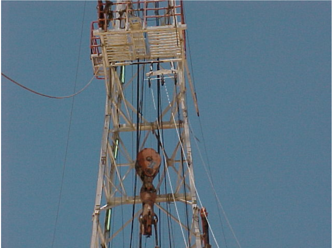
Figure 7.2 – Cable Sheaves Hanging from the Monkey Board
