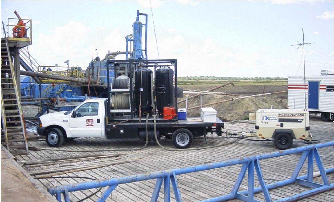
Figure IN2 – CP Unit with Compressor
